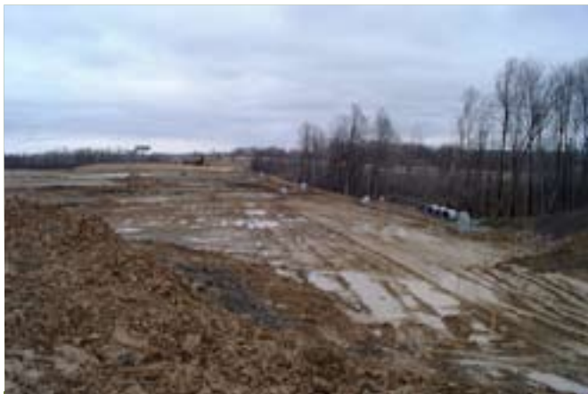
Portion of mass-graded 192 acre site;
