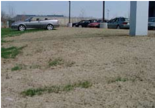
Silt Stop 740 Holds Mulch Over Winter - April 15, 2002
