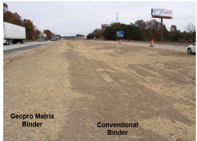
Geopro Matrix secured straw adjacent to west bound lanes
