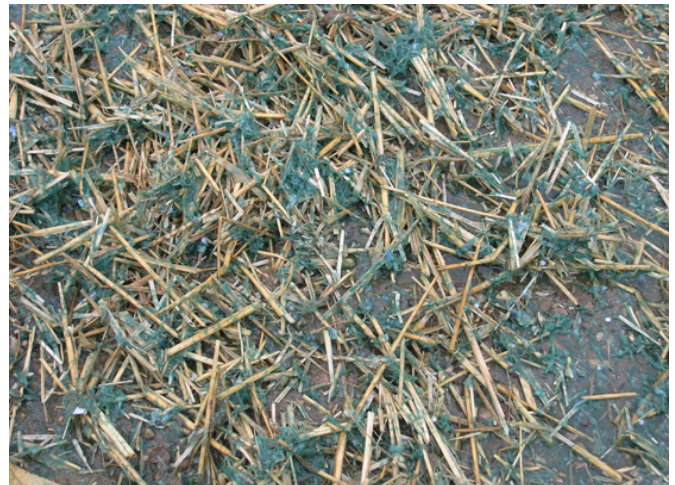
Geopro Matrix applied at 500-700 lbs/acre over blown straw
