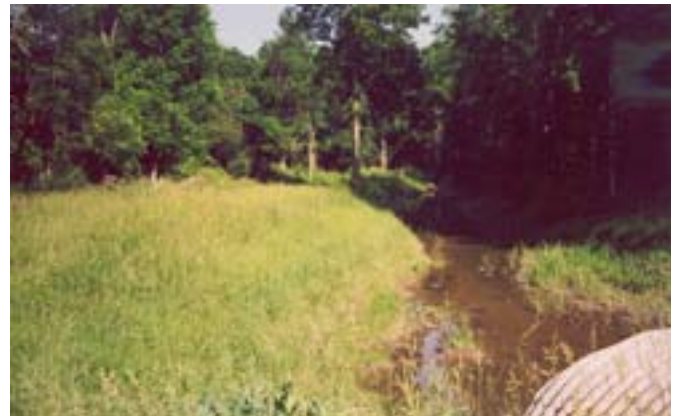
Dormant seeding using broadcasted Silt Stop 705 for soil binding
