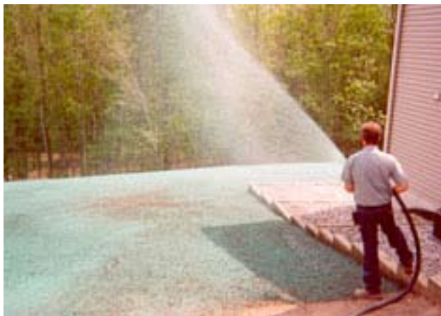
Applying Silt Stop 705 as the tackifier/soil binder within slurry
