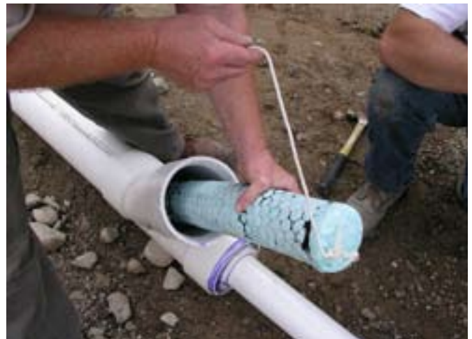
Insertion of 706b Floc Log into wye element
