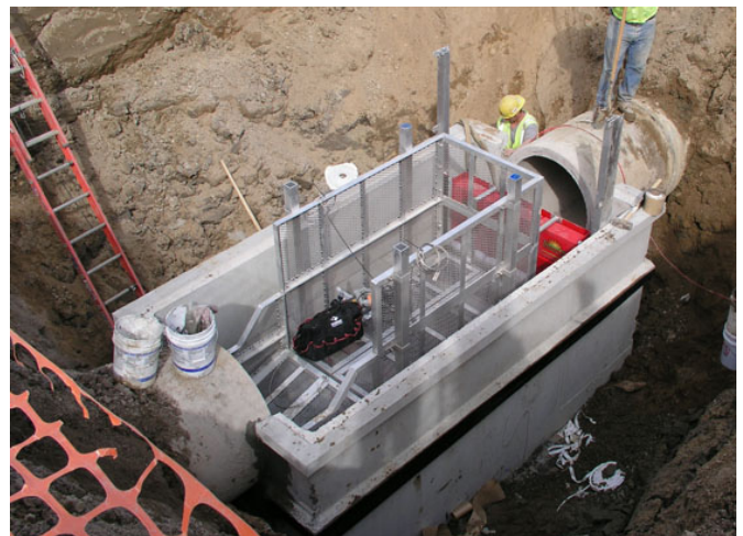
NSBB 6-12 unit retrofitted into 36" system
