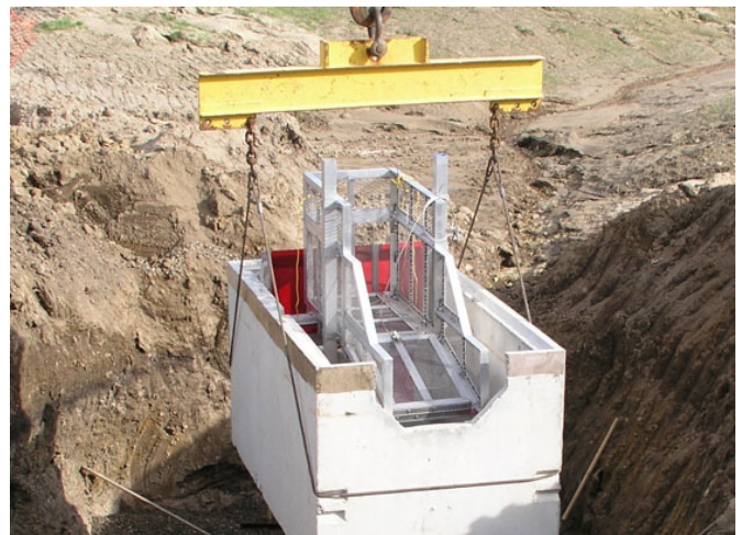
NSBB 4-8 bottom unit - screen systems are pre-installed at the plant
