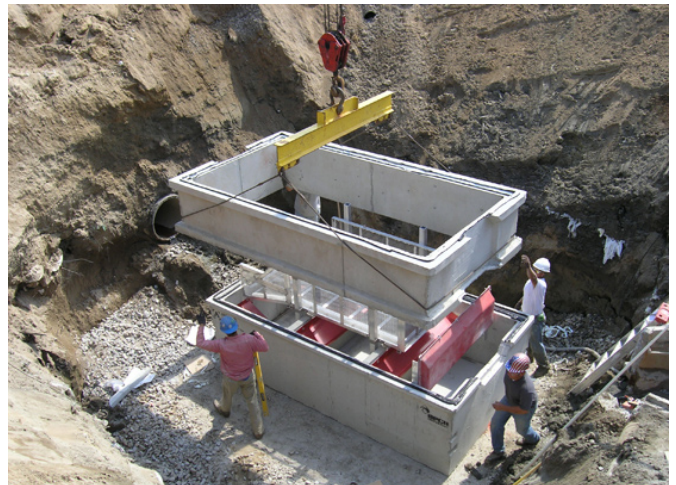
First mid-section being lowered into position
