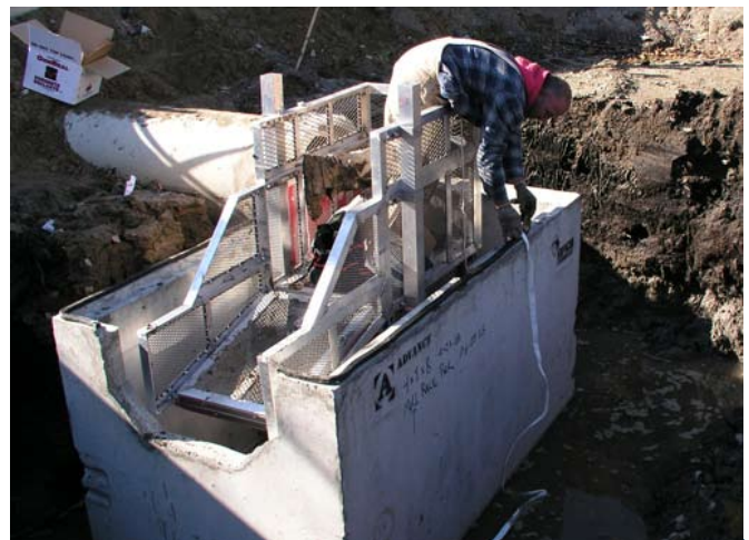
NSBB 4-8 unit - inlet pipe not yet installed
