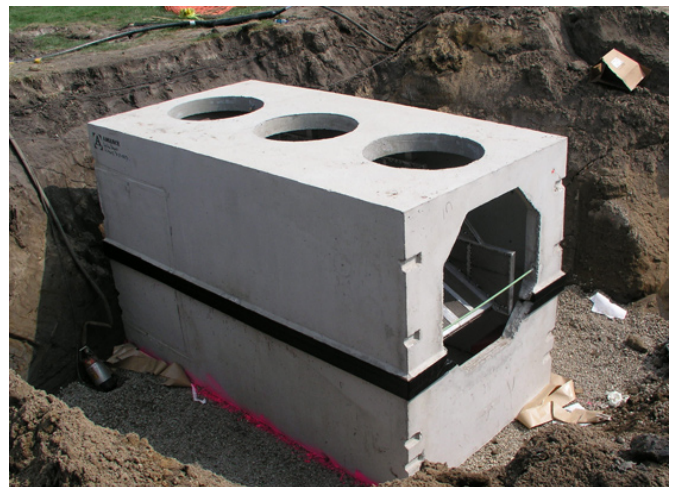
NSBB completed - ready for pipe installation & backfilling
