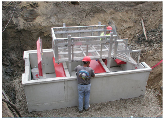
Bottom unit delivered to site with internal components installed
