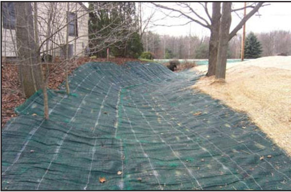
The P550 turf reinforcement mat provided the erosion protection needed in the channel.
