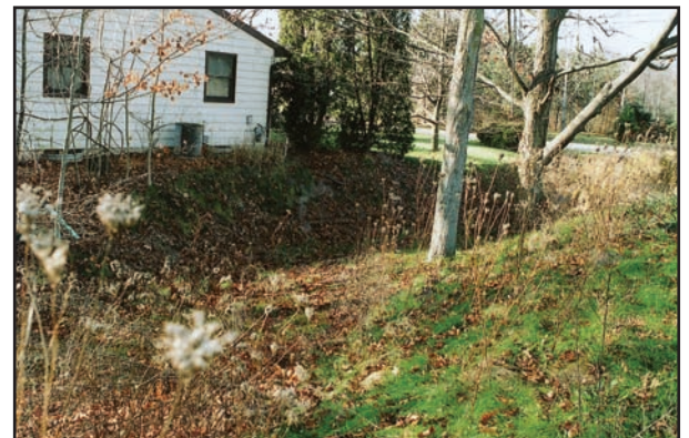
Within one growing season, the P550 had vegetated, leaving a natural channel bed that was pleasing to the nearby residents. The removal of the concrete also aided in easier maintenance and improved flow conveyance.
