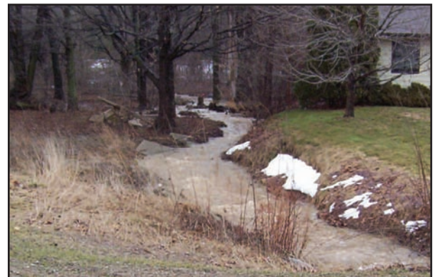
During heavy rain events, the large amounts of stormwater runoff flowing over the broken concrete slabs were creating unnecessary turbulence and added to the erosion process.
