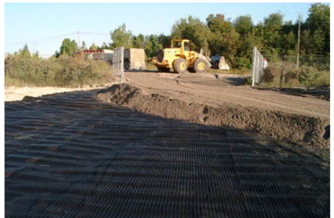
National Gypsum - Alpena, MI 2001 Propex 4553 Geotextile beneath Tensar BX1100 Geogrid
