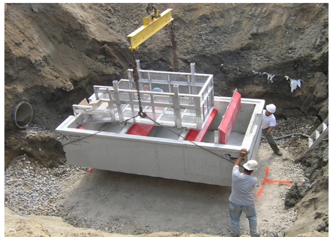
Knockouts are typically needed with larger pipe sizes
