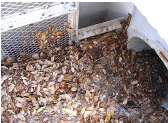
Leaves captured by NSBB screens - held above static water level
