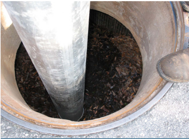
Vac truck removal of collected organic, debris & sediment
