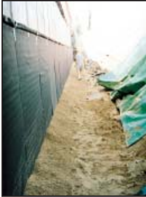
Wall Panel Installation
