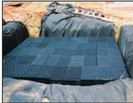
Approximately 1,000 cf of RainTank was installed at each residence.
