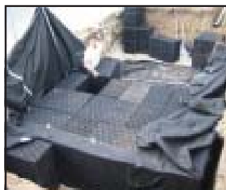
Placement of tanks.
