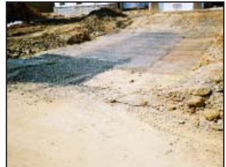
With only two feet of cover above the RainTank, a geogrid helps disperse the traffic load.
