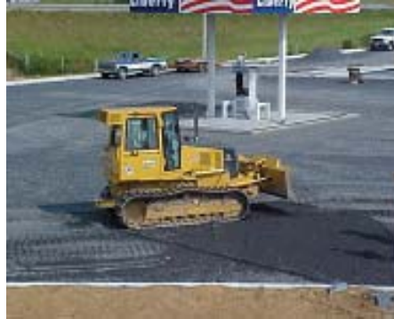
Most contractors use Low Ground Pressure (LGP) equipment to place cover materials.
