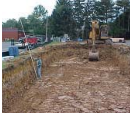
Excavation should be in accordance with all safety requirements.
