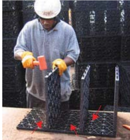
Build as shown. DO NOT use the rows of holes marked by arrows.
