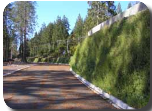
Vegetated Reinforced Soil Walls
