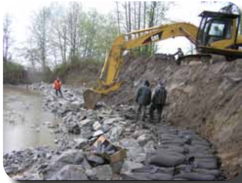
Over 1400 feet of shoreline was lost from erosion. Deltalok was used to form a permanent erosion resistant shoreline.
