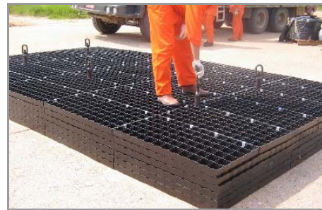
Figure 29: Assembling GEOTERRA™ Mats (Side-by-Side Pattern)
