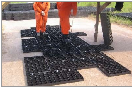
Figure 28: Assembling GEOTERRA™ Mats (Herringbone Pattern)
