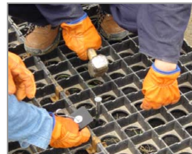
Figure 33: Driving the Anchor Head
