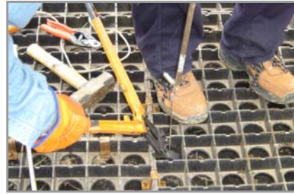
Figure 35: Crimping the Cable Stop
