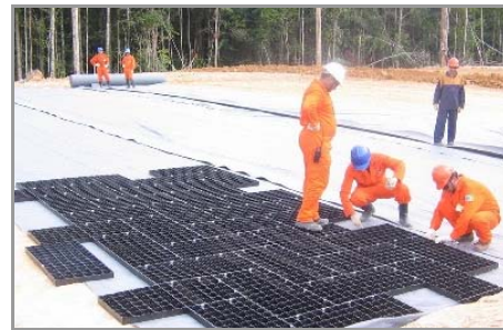
Figure 30: Placing GEOTERRA™ Mats Over Geotextile Layer
