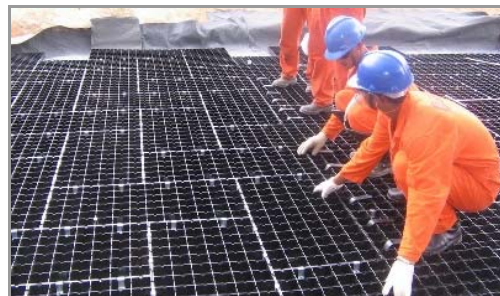
Figure 16: Connecting GEOTERRA™ Units
