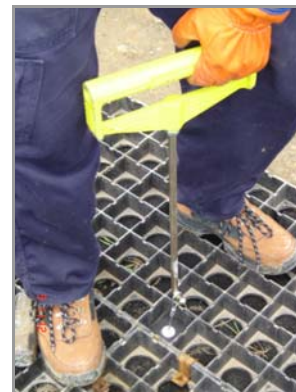
Figure 34: Setting the Earth Anchor
