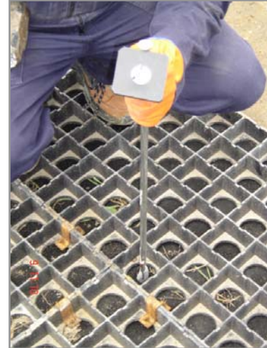
Figure 32: Installing the Earth Anchor
