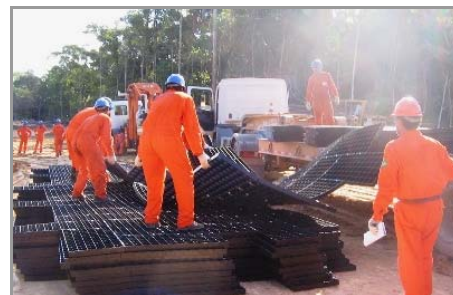
Figure 27: Transporting Pre-Assembled Mats from Off-Site
