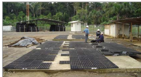
Figure 31: Connecting Pre-Assembled GEOTERRA™ Mats
