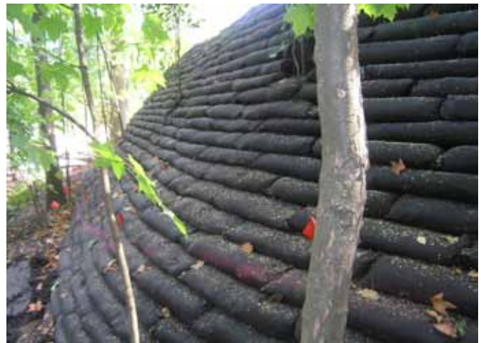
Picture 2: slope surface after bag placement
