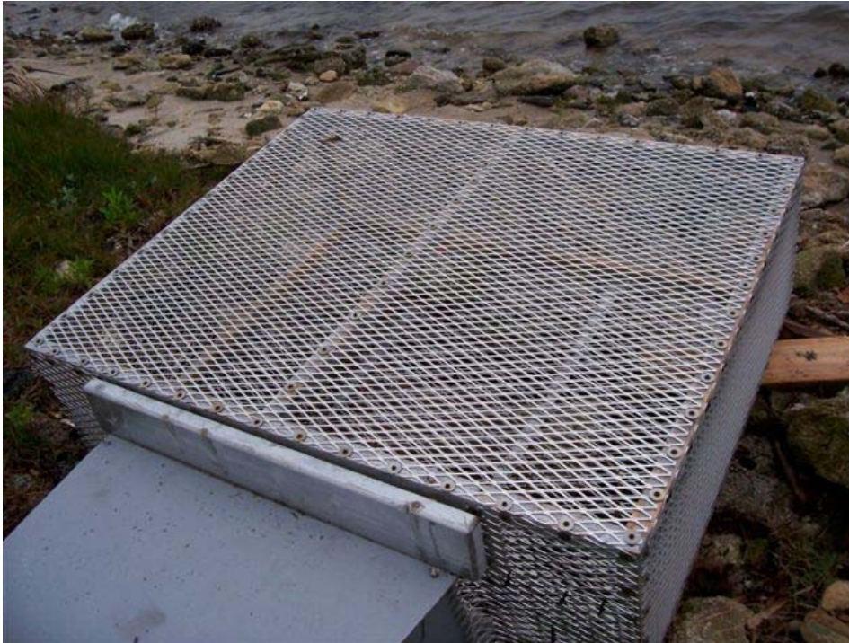
Figure 12. Effluent basket showing flume (2/12/2007).
