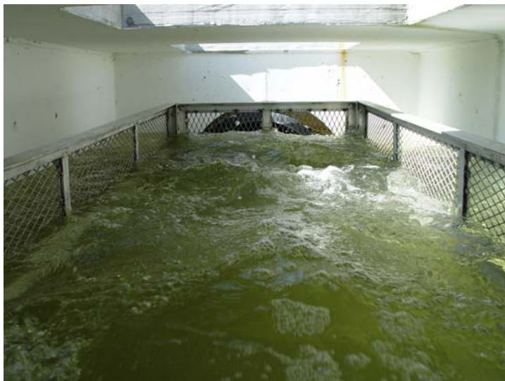
Outlet of Baffle Box at 9000 GPM
