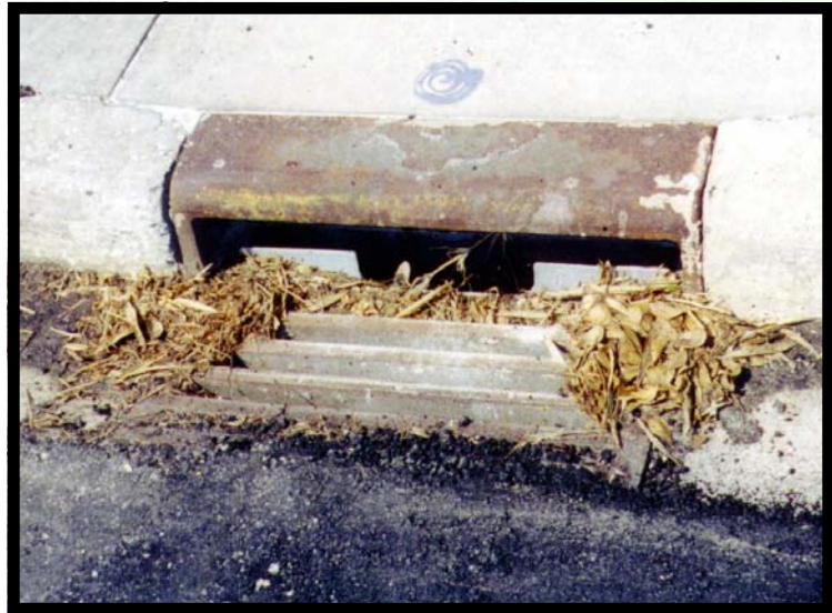
Above: View of inlet prior to any service work.
