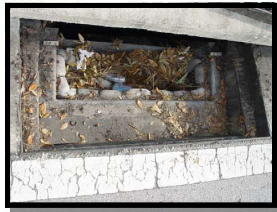
View of grated curb inlet immediately after the grate was removed.
